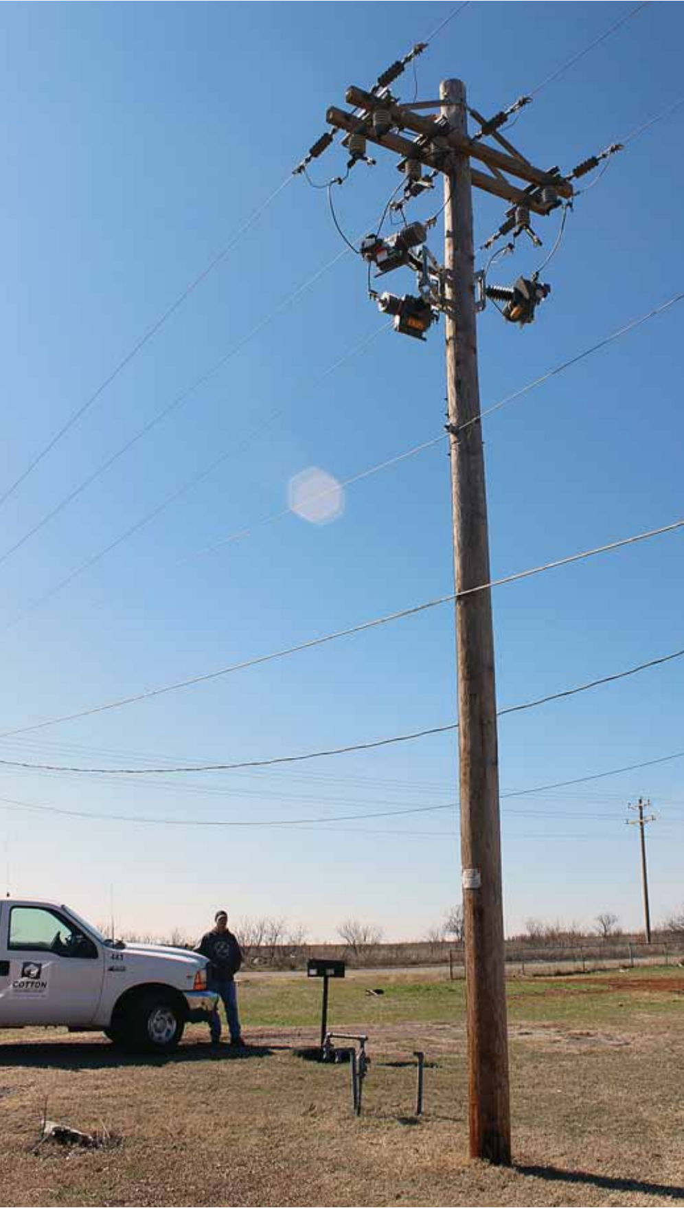
Devices on poles are larger than they appear, depending on the angle. A Cotton Electric vehicle and apparatus technician Zac Hoodenpile are dwarfed by this utility pole supporting three phases of power line and a trio of electronic reclosers.
