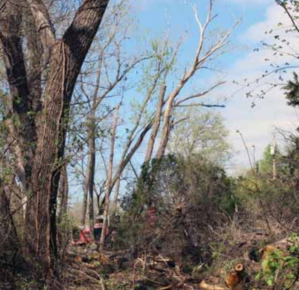
Contractors used a feller buncher recently to address a particularly overgrown wooded area that was causing power quality problems for Cotton Electric members. Many of the trees were dead and leaning toward lines; note the transformer on the right of the photos. The feller buncher made quick work of grasping the trees, cutting them at the base and stacking them to be mulched. The time elapsed in these before and after shots is 21 minutes.
