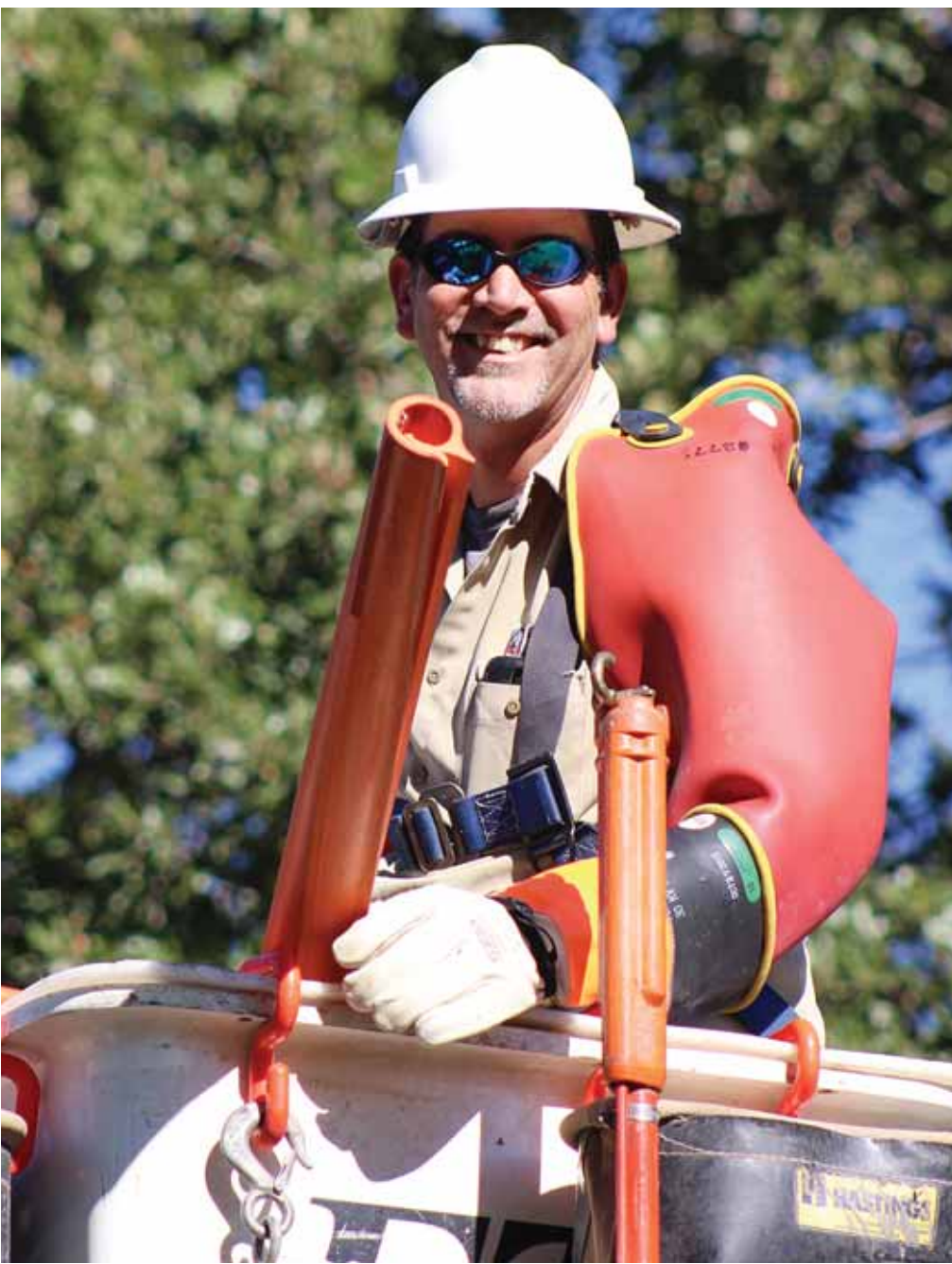
Jarrood Hooper has all personal protection equipment in place before raising up in a bucket to work on a transformer.
