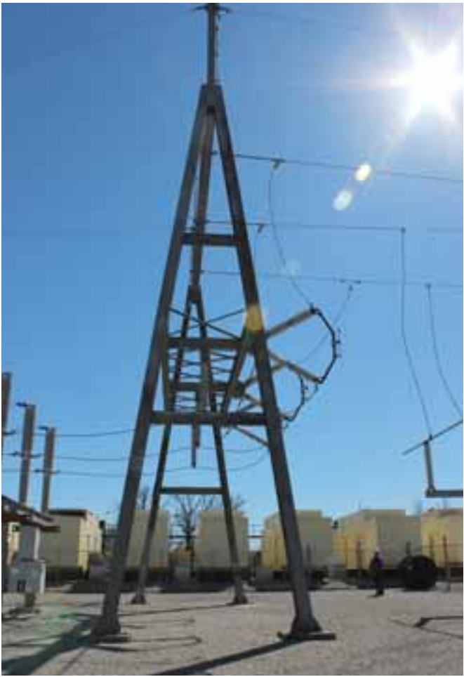
Two dedicated substations in eastern Stephens County are situated nearly side by side, separated only by a tall A-shaped metal structure where high voltage comes in from Western Farmers Electric Cooperative. The huge transformers of each sub step the electricity down to voltage useable at a nearby plant.
