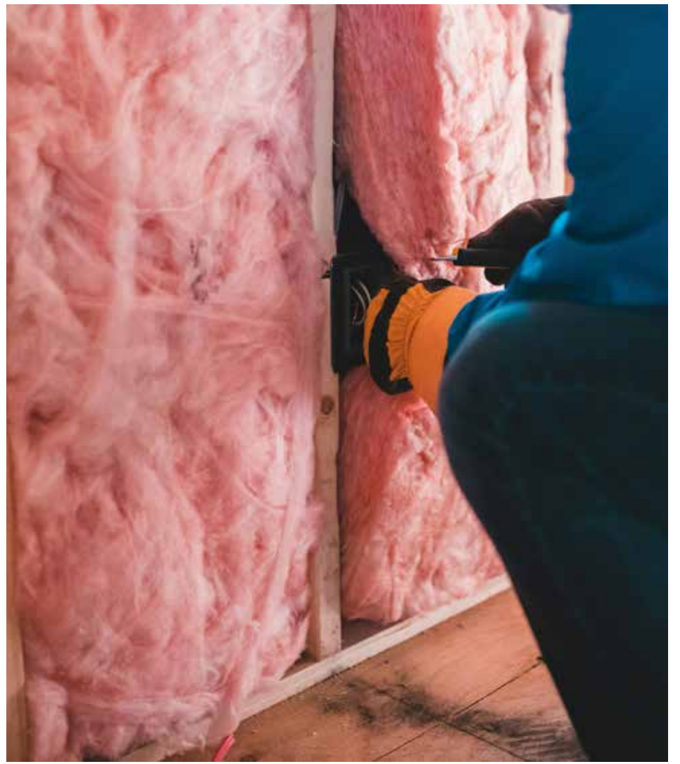
Installing proper insulation and air sealing around your home is an energy efficiency investment that enhances comfort while reducing energy consumption. Photo source: Erik Mclean.
