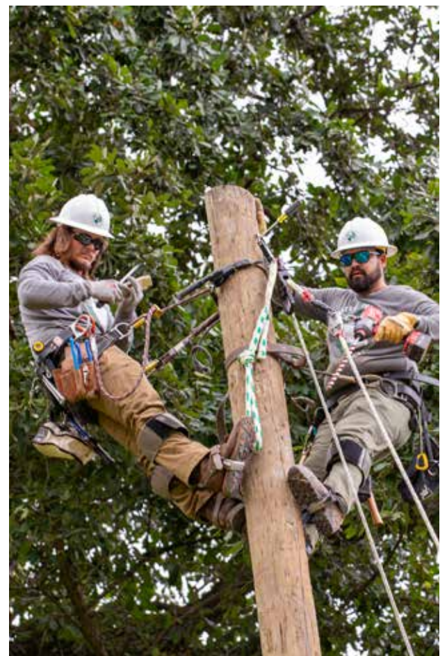
Hurst's (left) main responsibilities were framing and wiring poles. Photo courtesy of OAEC.
