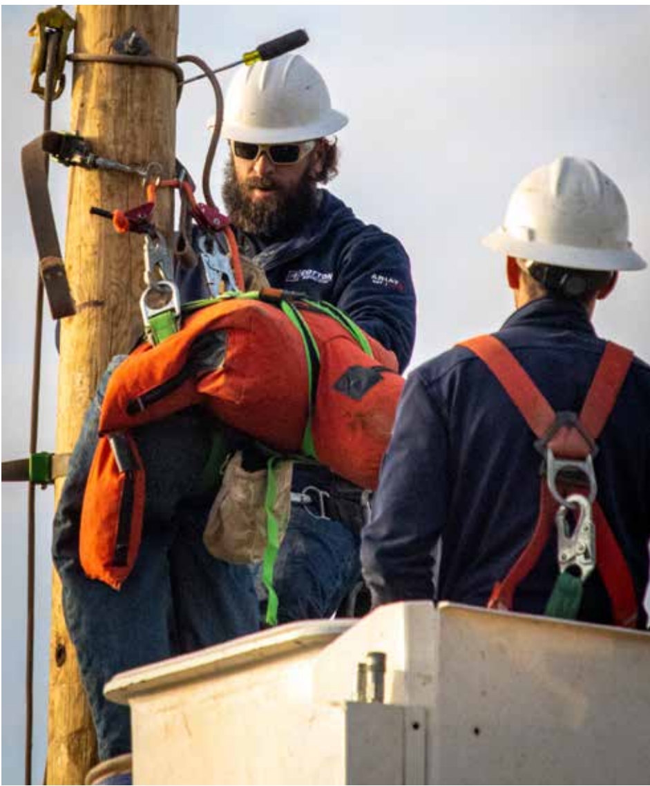
Cotton Electric Journeyman Lineman Marc Bohall completes his timed rescue. Photo by Carli Eubank.
